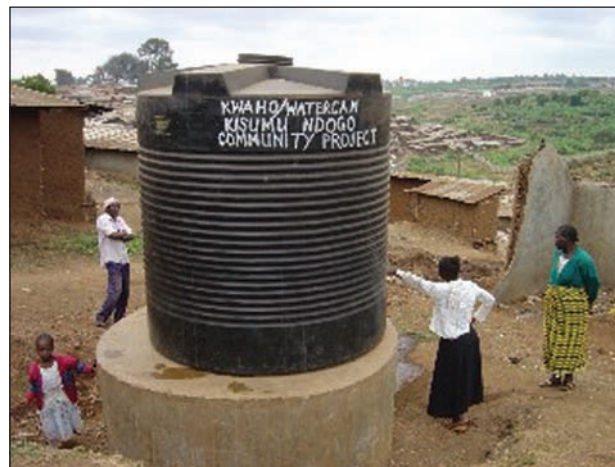
New, safe water storage tank
