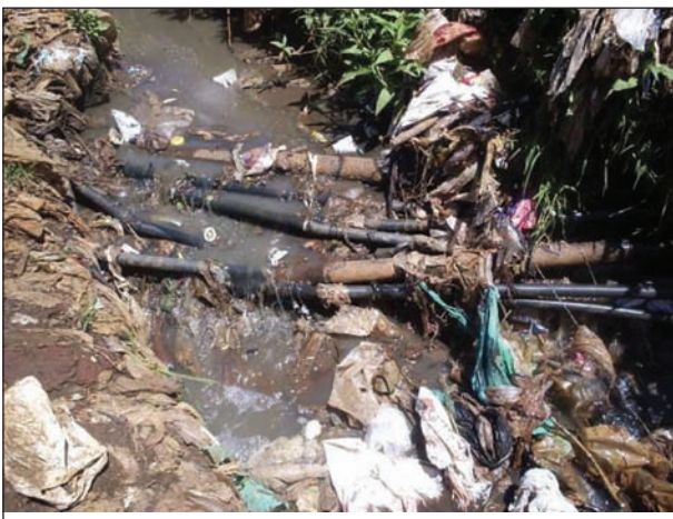
Old water pipes crossing a sewage trench
