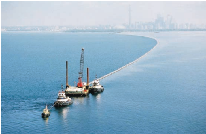
Figure 7 Toronto's water supply
